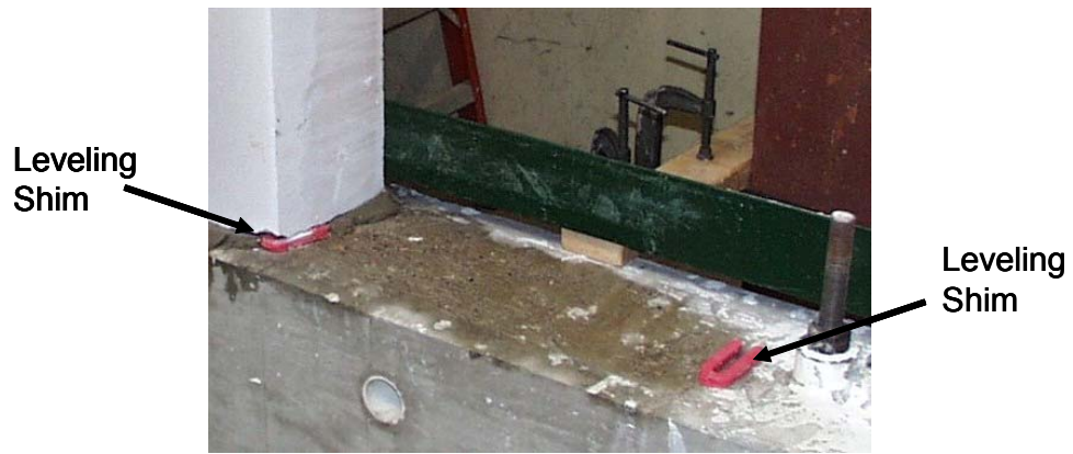
Figure 2.9: Preparing the foundation surface to place a vertical panel
