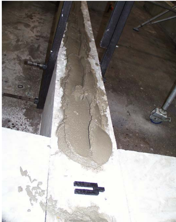
Figure 2.6 Placing Type S mortar by proportion on concrete foundation
