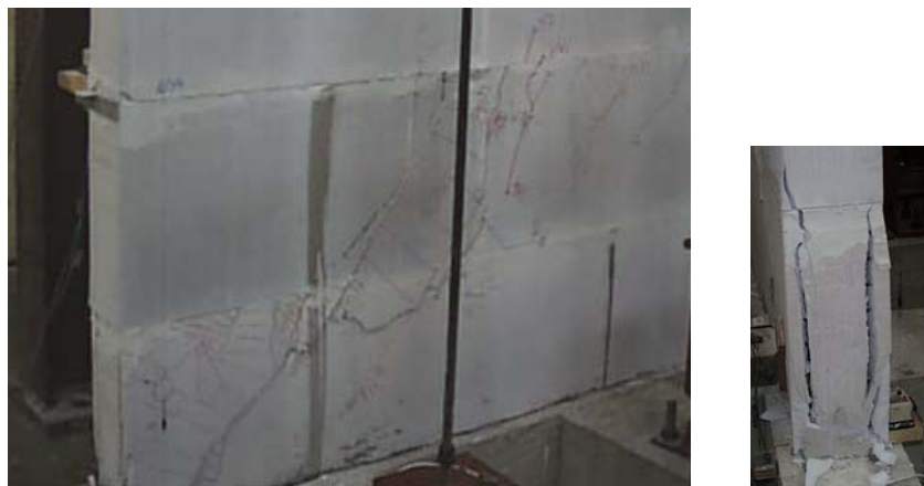
Figure 5.43: Front and side views of spalling at Load Point 871 in Shear Wall Specimen 4
