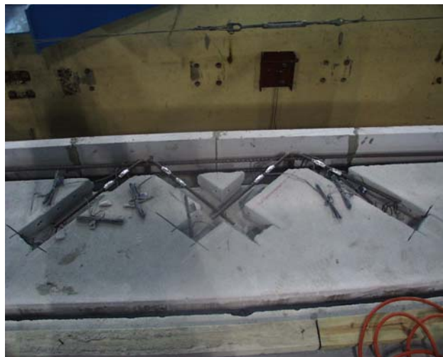
Figure 4.19: Picture of diagonal reinforcement across the joint parallel to the direction of load in Two-story Assemblage Specimen
