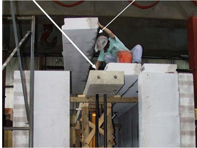
Figure 2.12: Placement of AAC floor panel in slab of Two-story Assemblage Specimen
