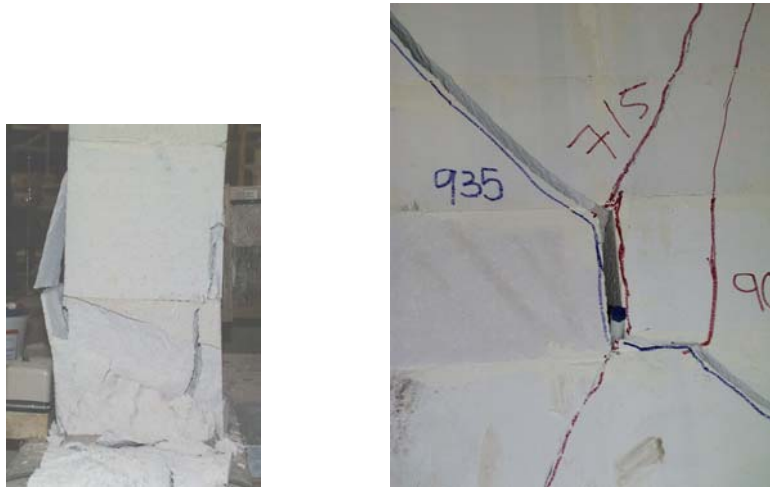
Figure 5.63: Toe crushing and opening of web-shear crack in Shear Wall Specimen 7
