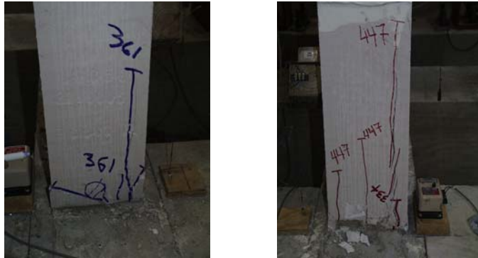
Figure 5.69: Vertical cracks at the base of the south and north ends of Shear Wall Specimen 9
