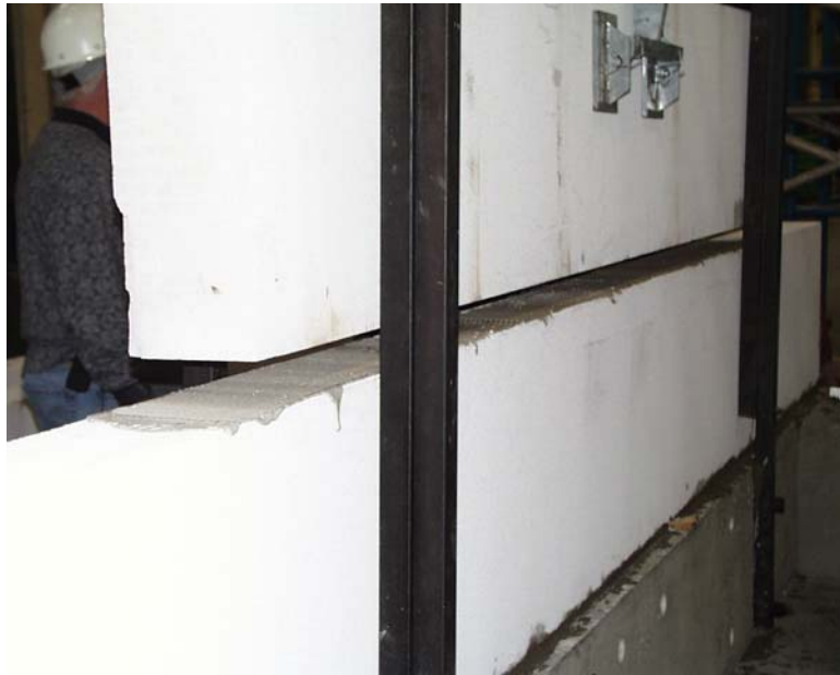
Figure 2.8 Placing second course of AAC panels in Shear Wall Specimen 1
